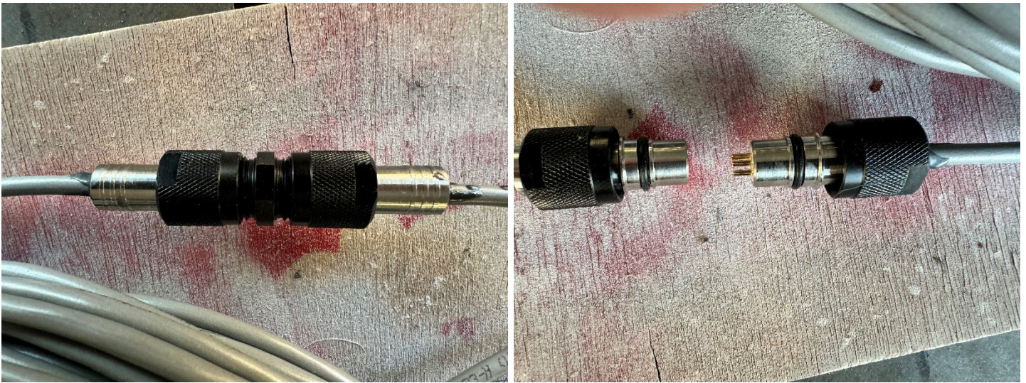
Figure 16: New connector installed and utilized.
