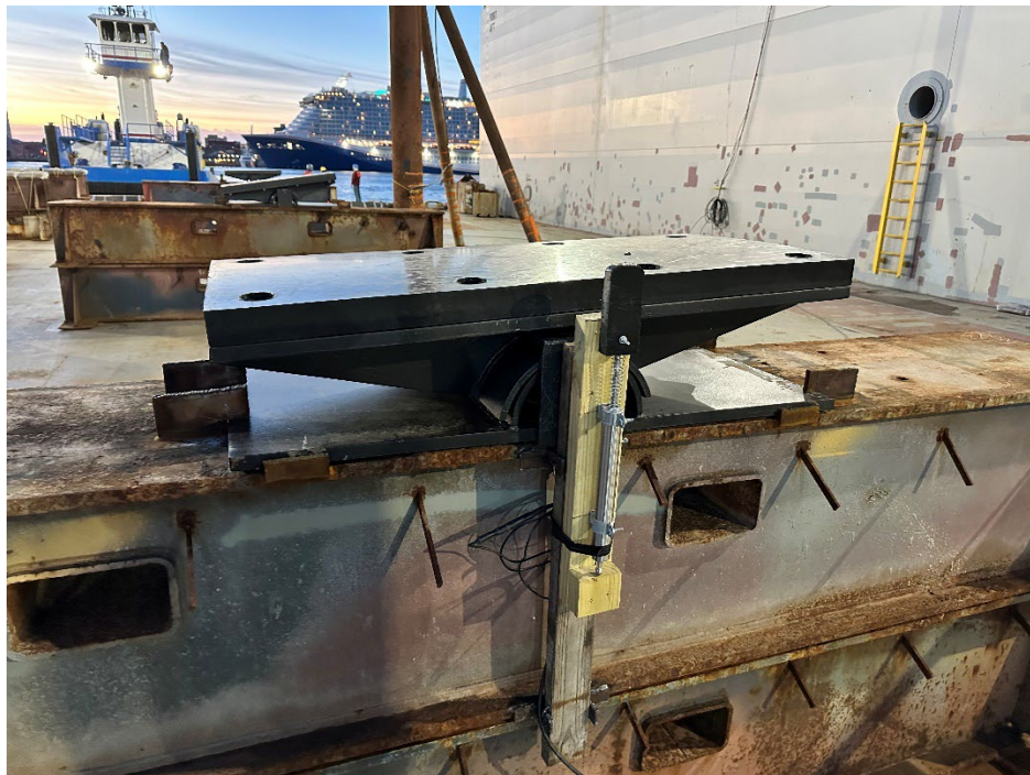
Figure 13: Docking 3 HDPE Side Block Before Docking
