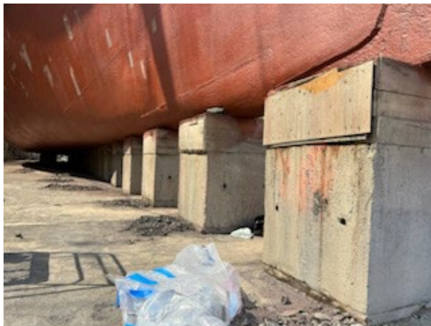
Figure 19: Old Fiber-Reinforced Concrete block under a USCG Cutter.
