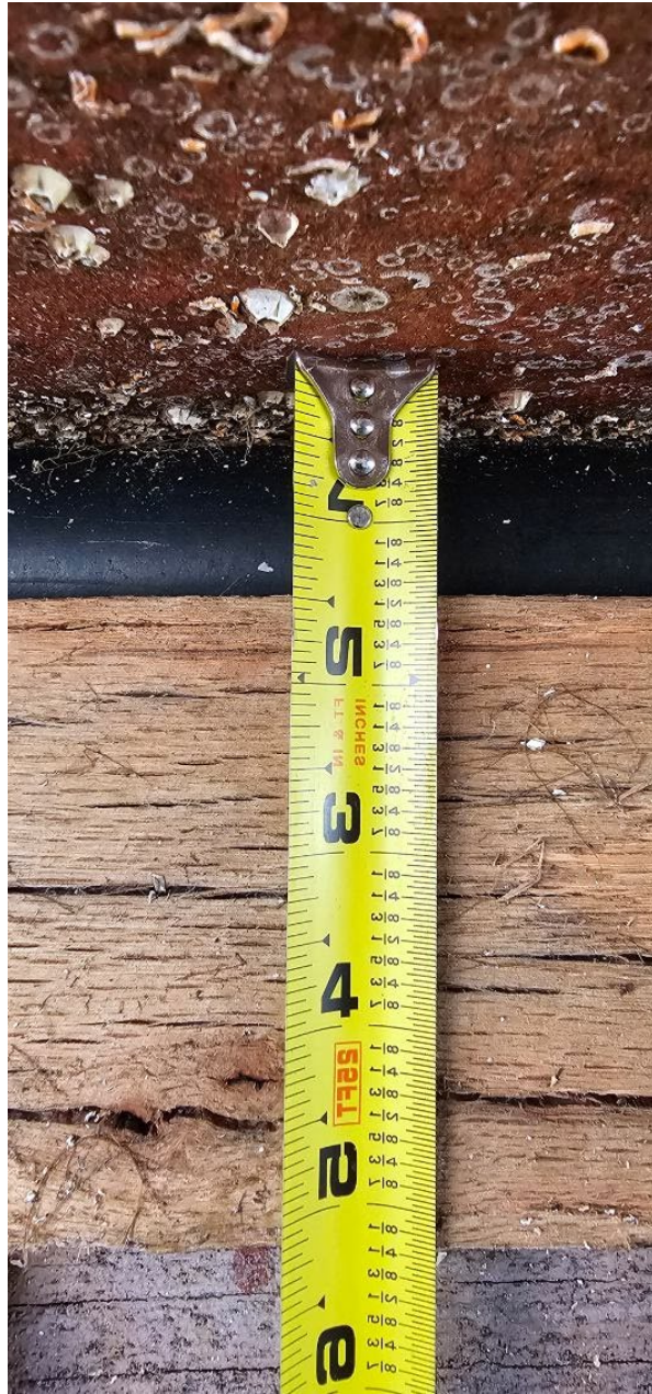
Figure 8: Docking 2 Neoprene Side Block Loaded Showing 1/2" Compression
