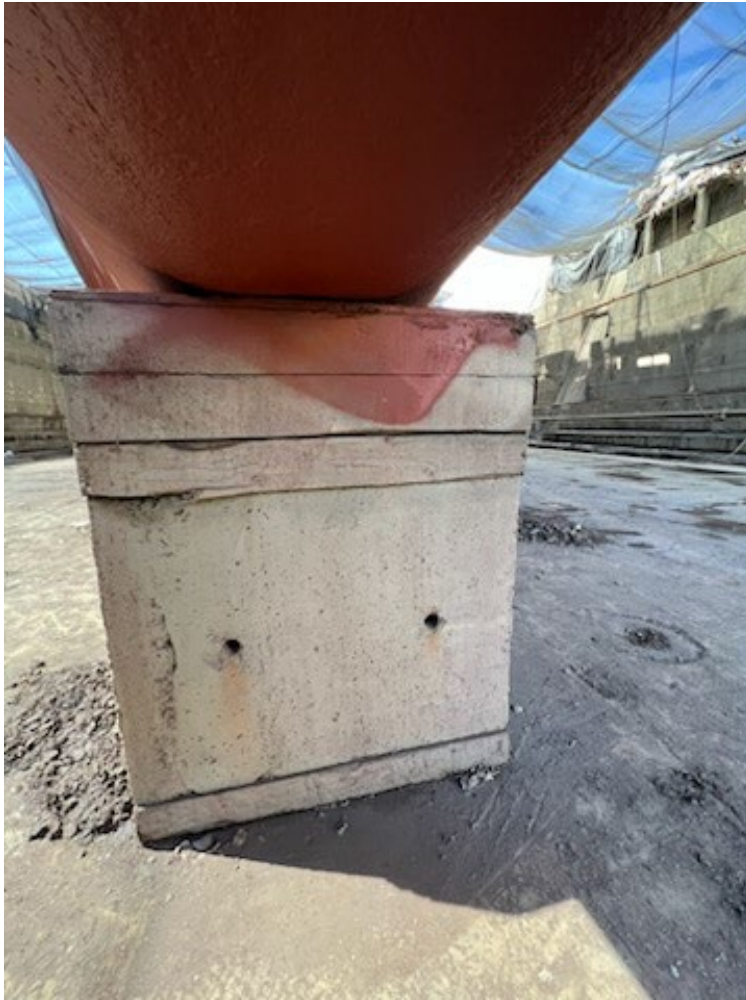
Figure 16: (old) Fiber-reinforced block under USCG Cutter
