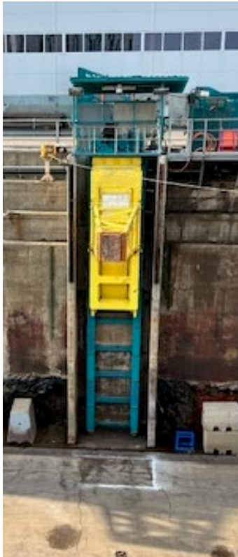
Figure 9: Photo of Sidewall Support Lifting Track
