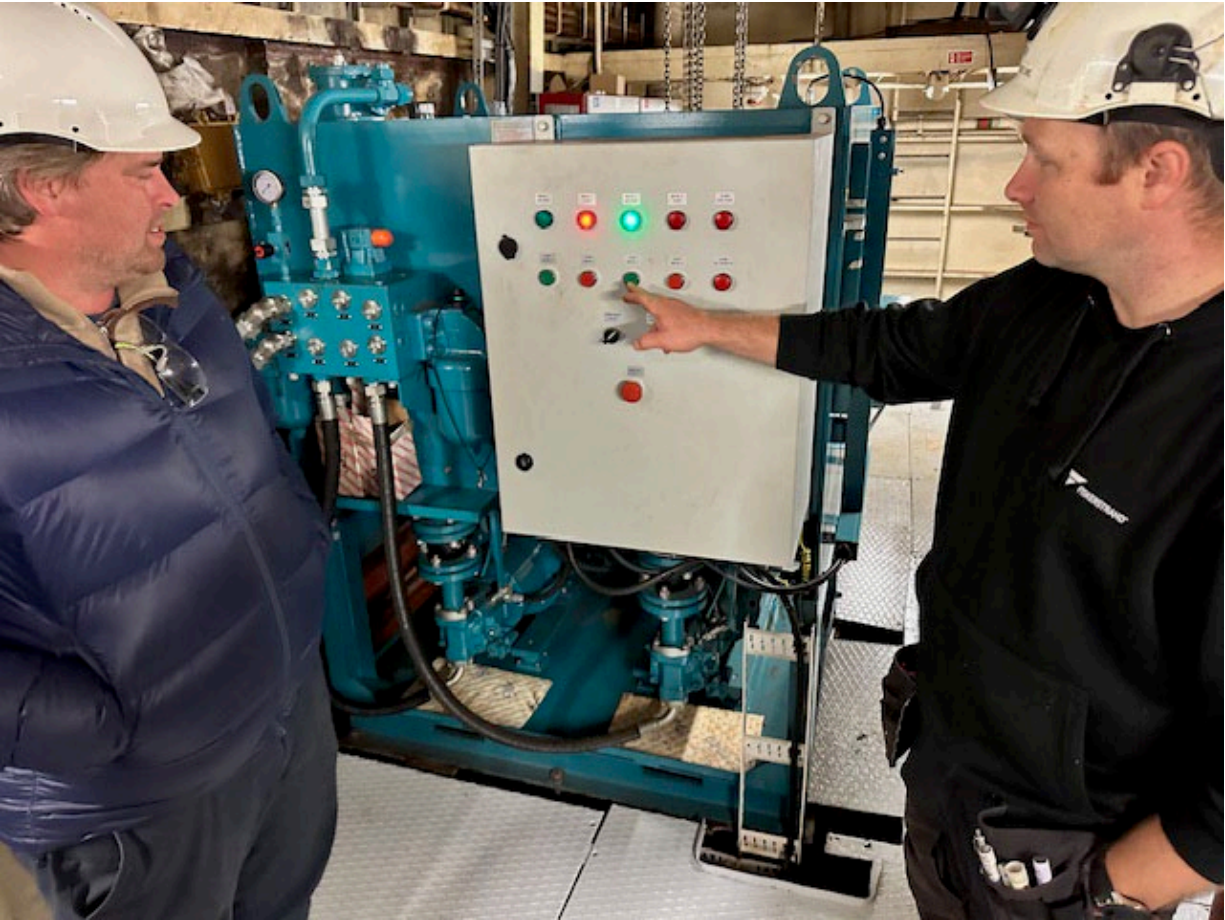
Figure 5: Photo of Bilge Support Arms HPU
