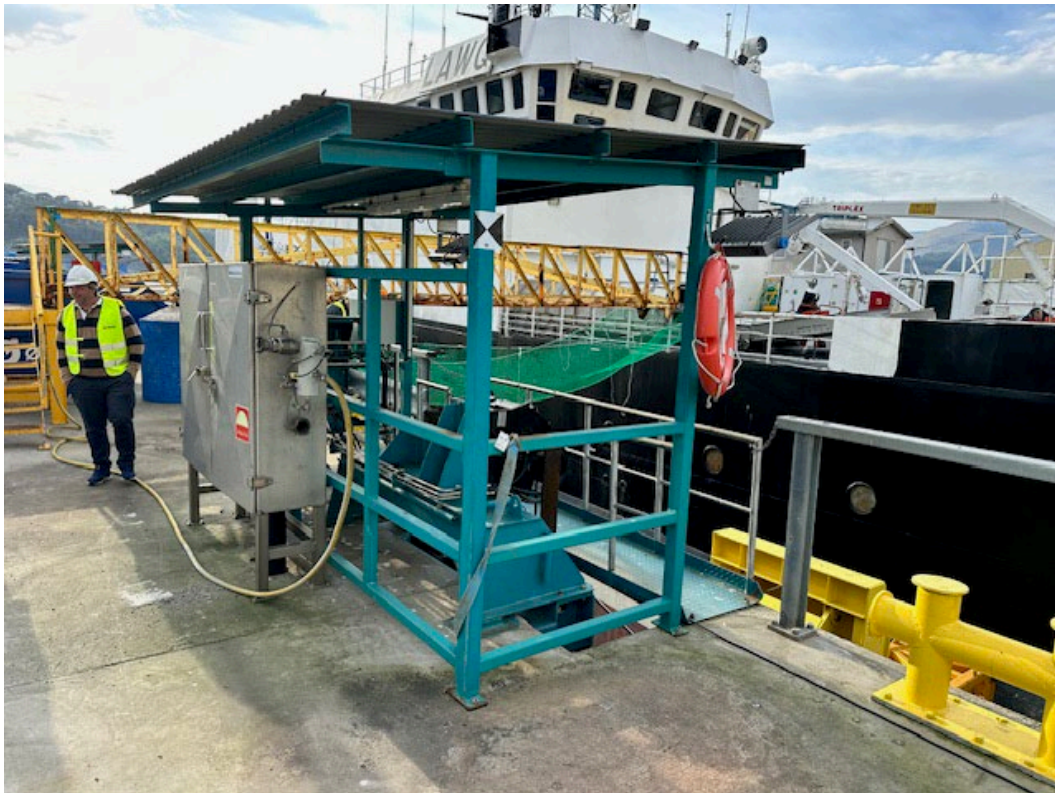
Figure 10: Photo of Sidewall Support Lifting Mechanism
