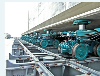
Venice Mose project, Caisson, Transfer System
